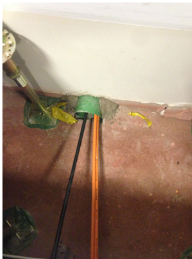
Internal Access at
